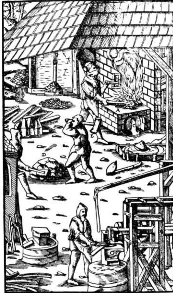
Figure 17. Iron-smelting furnace and forge, mid-sixteenth century.
